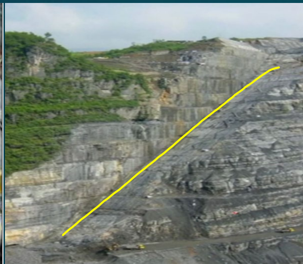
趾板基础开挖
