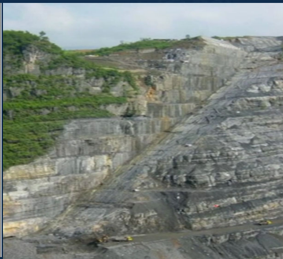
趾板基础开挖
